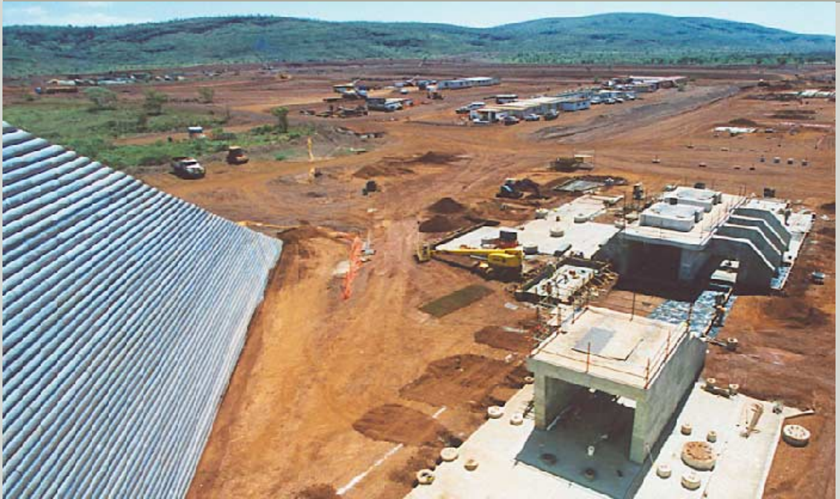
Picture: Foundations for Area C crusher
