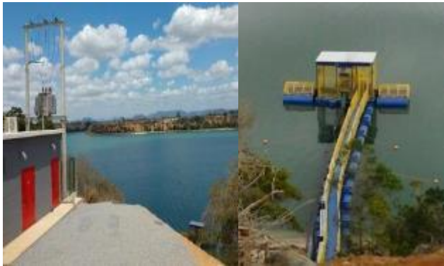
Lagoa Nova pipeline in Linhares
