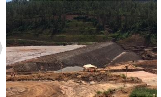
Rebuilt Santarem Dam, March 2016
