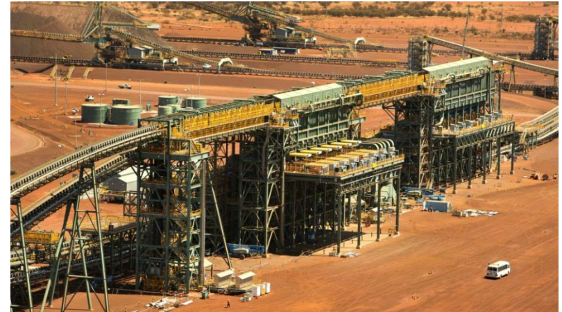
Jimblebar ore handling plant
