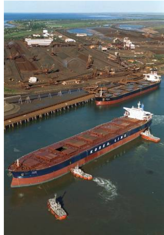
Port Hedland, Australia
