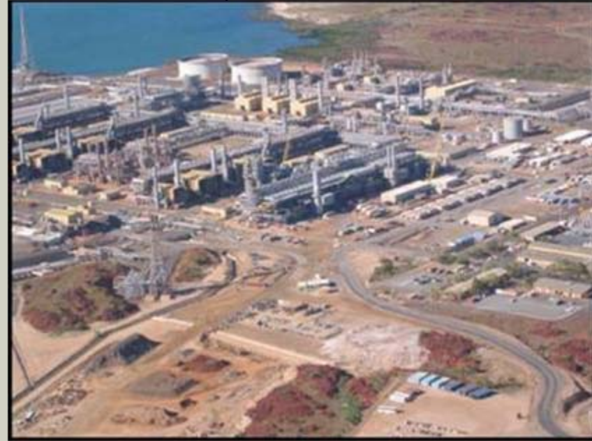
Onshore Gas Plant pre-Train 5
